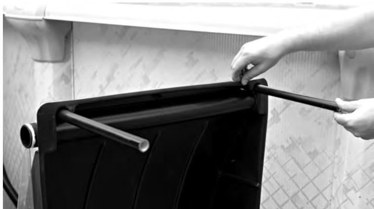
5. Wrap ample amounts of Teflon tape (provided) on the ends of all four threaded headers and pipe adaptors.
