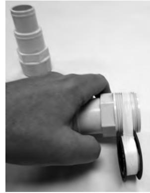
6. Thread pipe adaptors to 1½" pvc coupling. Attach coupling and pipe adaptor to front/lower headers. Hand tighten, then use a channel lock to further tighten by a half-turn.
