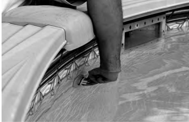
9. Make sure filter is turned off so no water flows out of the filter when disconnecting return hose from the swimming pool return and connecting to the SolarArc.
