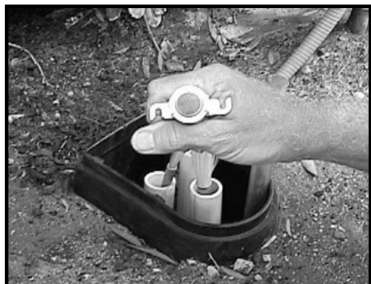
10. Inspect the cut, no lines or "puddles".
