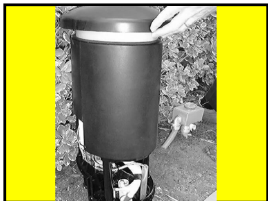
14. Carefully install outer body.
