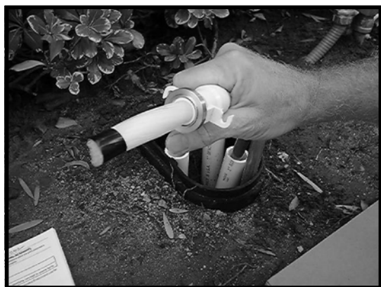
8. Screw on the cutting shield.
