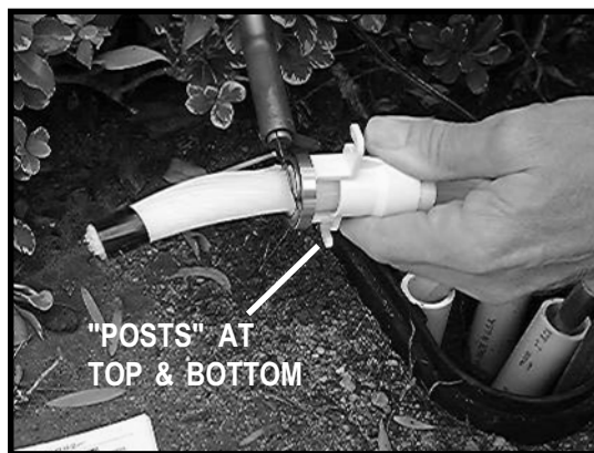
9. Hot knife cut, at a 15 deg. blade angle.
