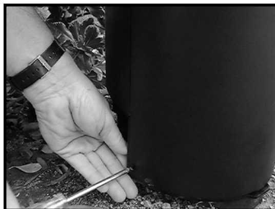
15. Secure outer body with two screws.
