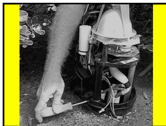
13. Secure PG2000 to base with 4 screws provided.
