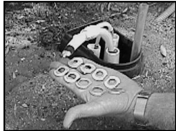
6. Select the correct "numbered" fiber disk.
