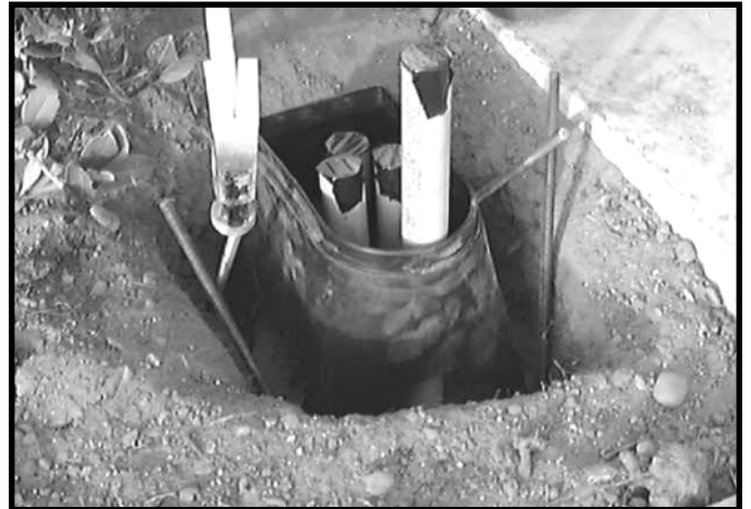
3. Drive 3/8 in. rebar at an angle in the corners.
