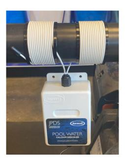
This is what it should look like after installation. Note that the left hand wire goes under the plastic tie and over the top of the pipe with a second plastic tie securing the end. The right hand wire goes under the pipe and under the plastic tie and winds in the opposite direction.
