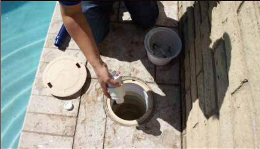
7. Connect **the elbow connectors (#18)** to each other so they angle the hose out the skimmer door, then slide the female end over the top of the Automatic Regulator Valve.
