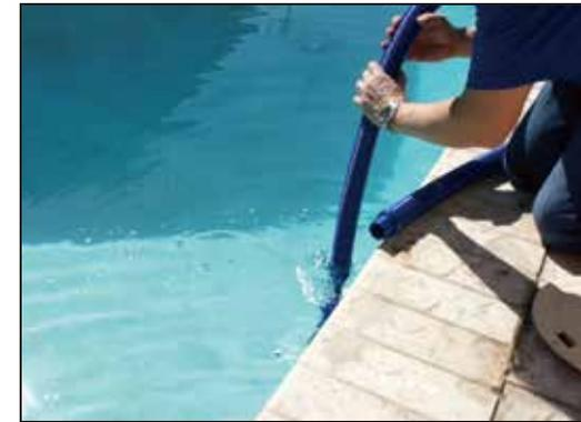
**TROUBLESHOOTING TIP:** If the return line pushes the cleaner away from that area of the pool, adjust or install an eyeball diverter.
