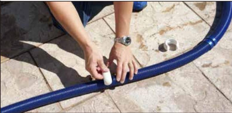
3. Place the **hose weight (#17)** on the hose. You will need one hose weight if your pool depth is less than 8 feet, two if the pool depth is more.
