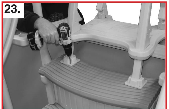
Using a cordless drill/driver attach the two mounting blocks to the pool step using eight [8] #10 x 1-1/4" screws. Secure the adjustable tubes to the adjustable tube handrail at the pre-marked locations using two [2] #10 x 1-1/4" screws in each handrail.
