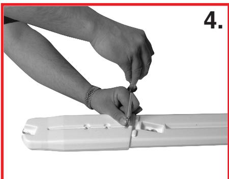
4. Using two 1/4-20 x 2" long bolts and two acorn nuts fasten the extension boots to the ladder legs
