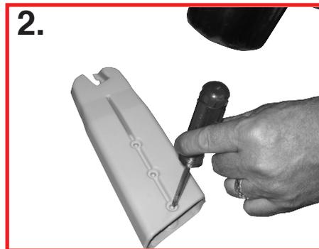
2. **Extension boots are not required if the outside height of your pool (measured from the ground to the top of the pool ledge) is 48" or less. If this measurement is more than 48" extension boots will be required.** Using a Phillips screwdriver tap out the plastic film from the top hole on each side of the extension boots.
