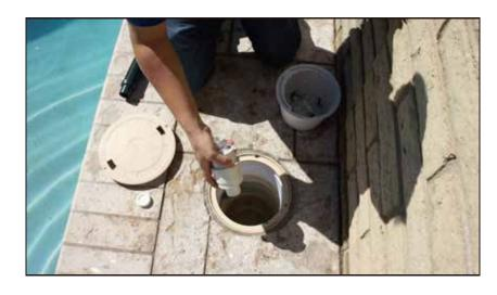
7. Connect **the elbow connectors (#18)** to each other so they angle the hose out the skimmer door, then slide the female end over the top of the Automatic Regulator Valve.
